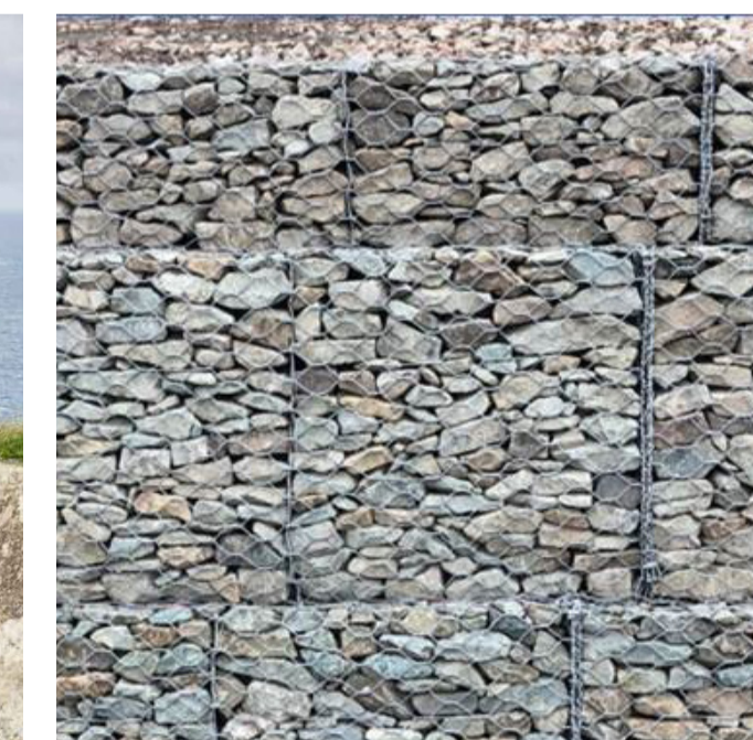
Stone faced welded mesh gabion wall
