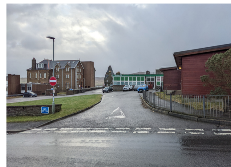
Site entrance from Lover's Loan
