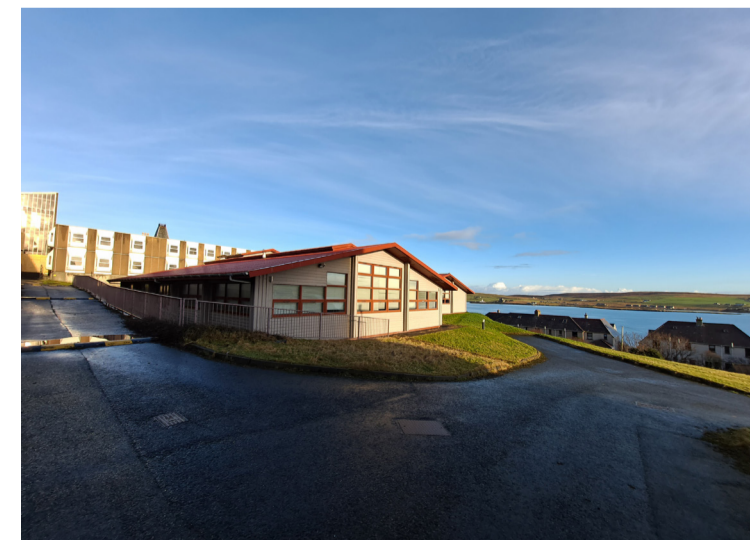
Former Science Building from Gressy Loan
